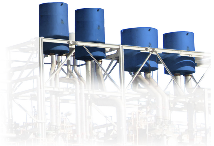
Vent Silencer Array at a Power Plant
